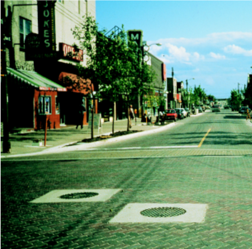
Figure 7. Concrete collars protect utility structures.
