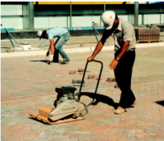
Figure 10. A plate compactor seats the pavers in the bedding sand.
