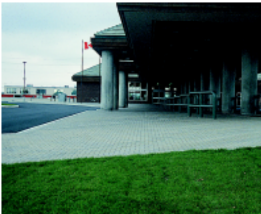
Figure 14. Success breeds success: concrete pavers at the North Bay train station.
