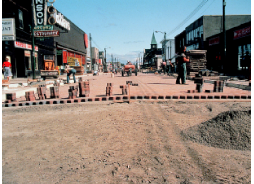
Figure 9. A crown in the road contributes to interlock by allowing the pavers to settle and tighten slightly under traffic.
